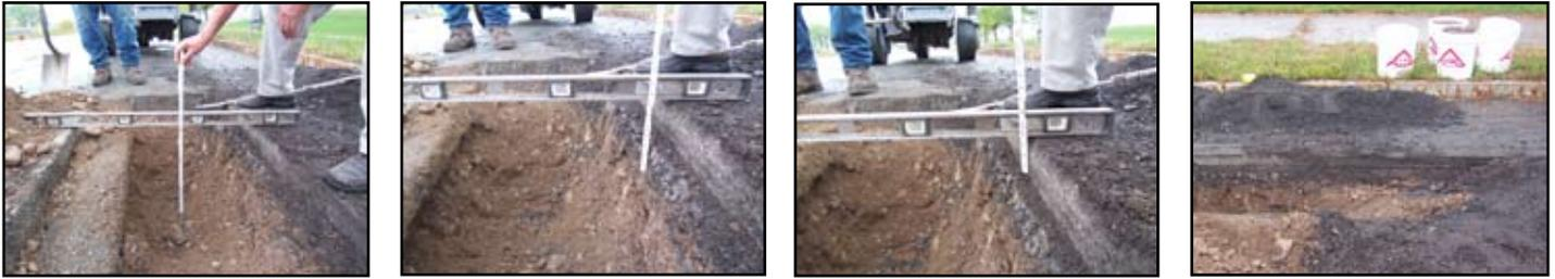
Asphalt pavement was removed to a depth of 4" by milling. Millings were stockpiled in an adjacent parking lot and supplemented by other Xerox milling. Shoulder excavation was removed along with 2 feet of the existing pavement edge to accommodate new under drain system and to accommodate new shoulder sub base material. This excavated material was not suited for recycling as it contained silts and organics.
