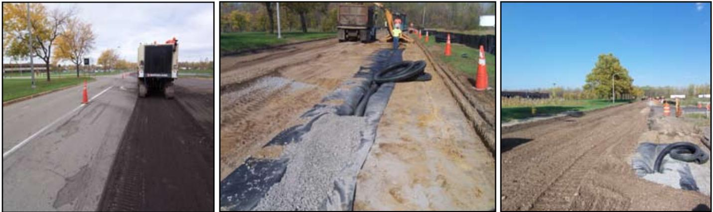
Remainder of the asphalt and sub base materials were dry recycled to provide a free draining sub base material for the roadway and shoulder section. Sub base material was graded and recompact in preparation for paving. Roadway was open to traffic during this construction.
