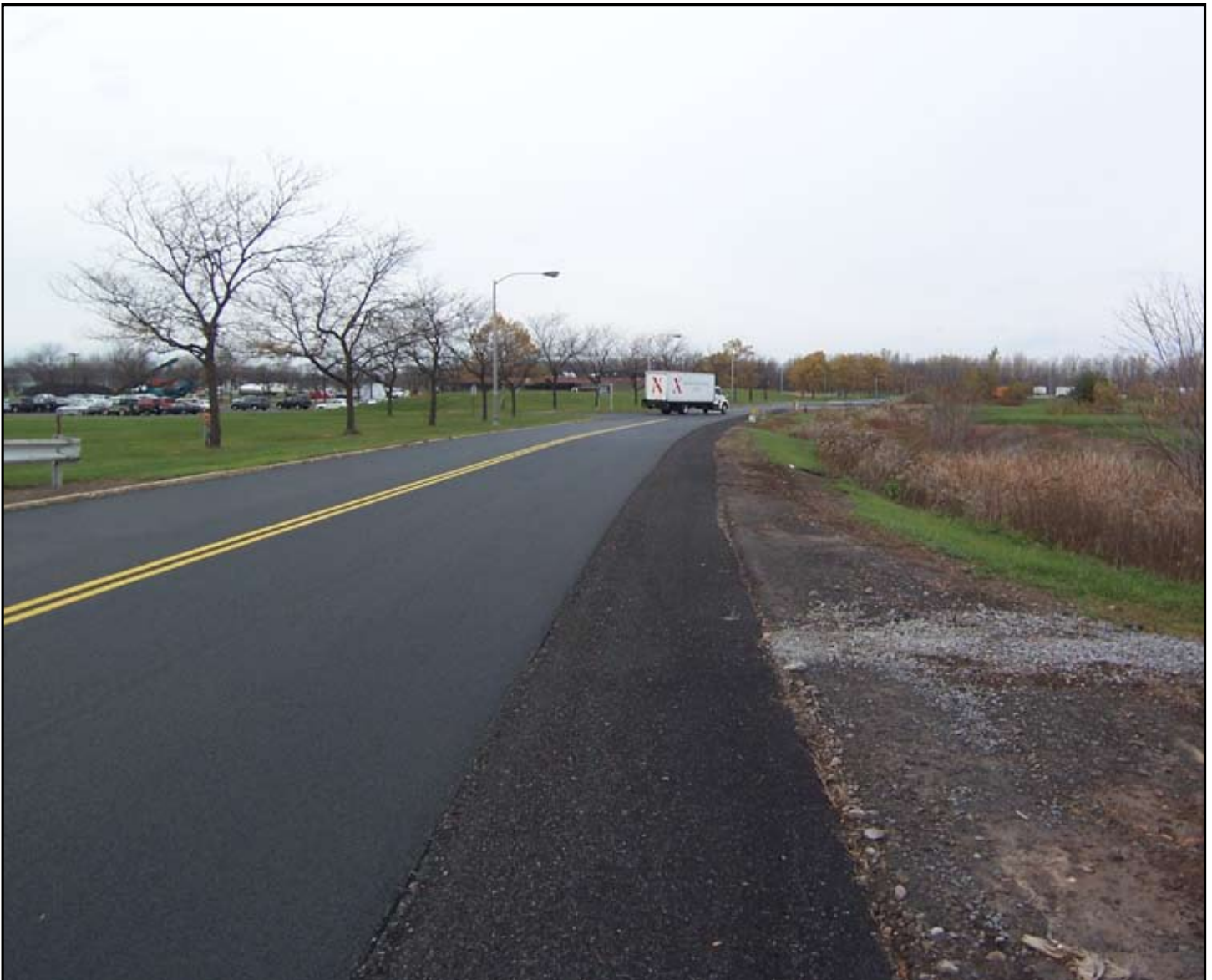
Resende Drive / Post Construction
