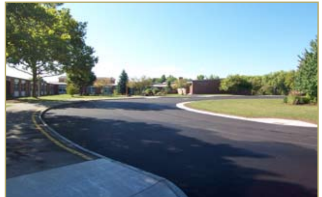
State Road Elementary School Bus Loop
