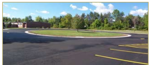
Klem Road Elementary School Bus Loop
