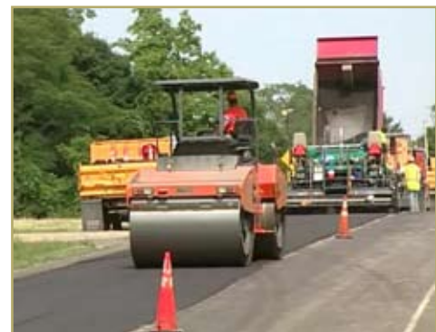
Paving Lake Road with SmartPave
