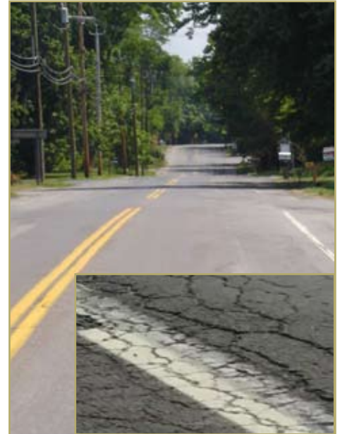
Lake Road prior to reconstruction
