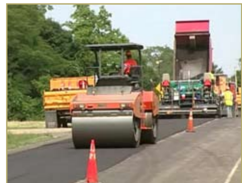
Paving Lake Road with SmartPave
