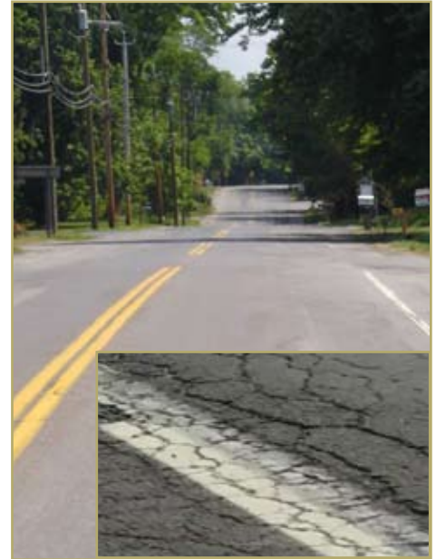
Lake Road prior to reconstruction
