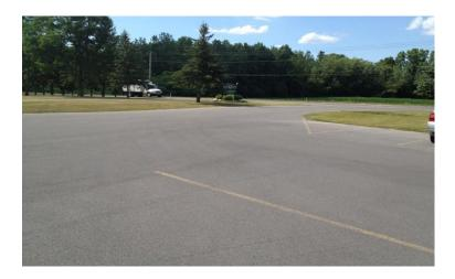
**Comments:** Existing parking lot and entrance road was crushed stone. Area was graded and recompacted. 3" FoamMaster® recycled base was paver placed followed by  $1\frac{1}{2}$  inch Hot Asphalt top.
